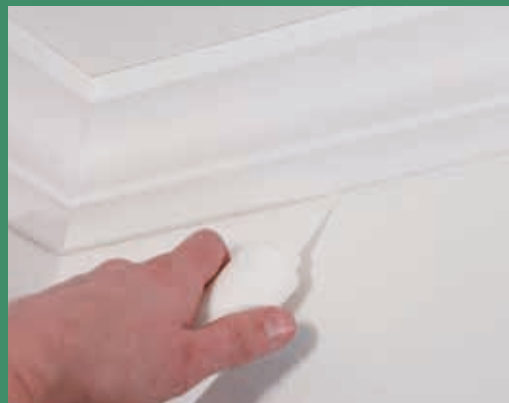
Sealing of wall joints
