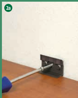
Drilling of the holes for the CH23 clipholders for profile heights of less than 90mm/3-17/32" with a drilling template
