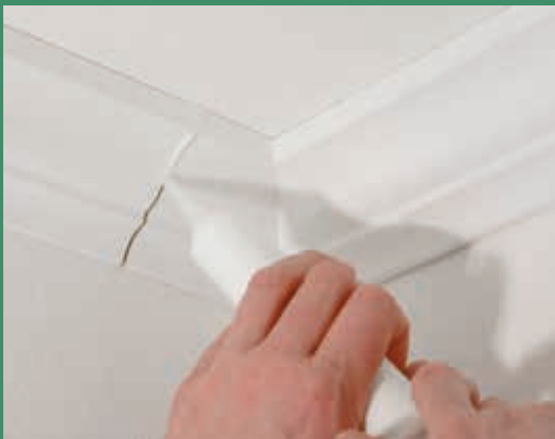
Sealing of expansion joints
