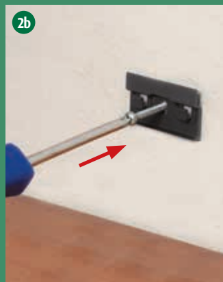
Drilling of the holes for the CH23 clipholders for profile heights of more than 90mm/3-17/32" with a drilling template
